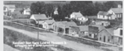
Looking northeast from the Mondamin's north elevator in 1906.
